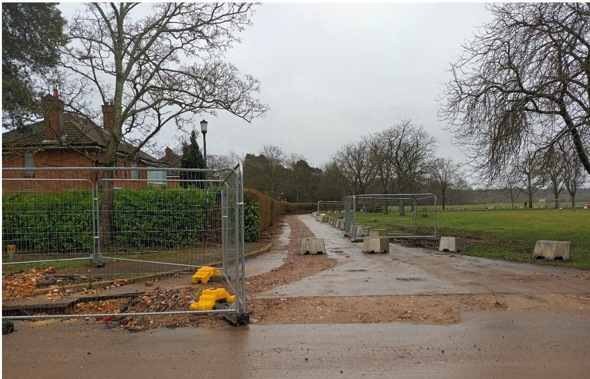
VIEW FROM SOMME ROAD TOWARDS FORMER MILITARY ACCESS ROAD (NORTHERN END)
